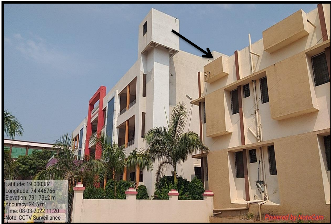
Picture 2: CCTV Surveillance System at Rajmata Jijau Girl's hostel
