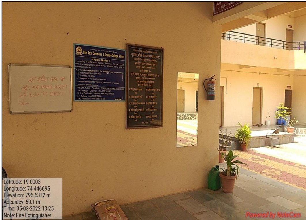
Picture 9: Fire Extinguisher at Rajmata Jijau Girl's hostel
