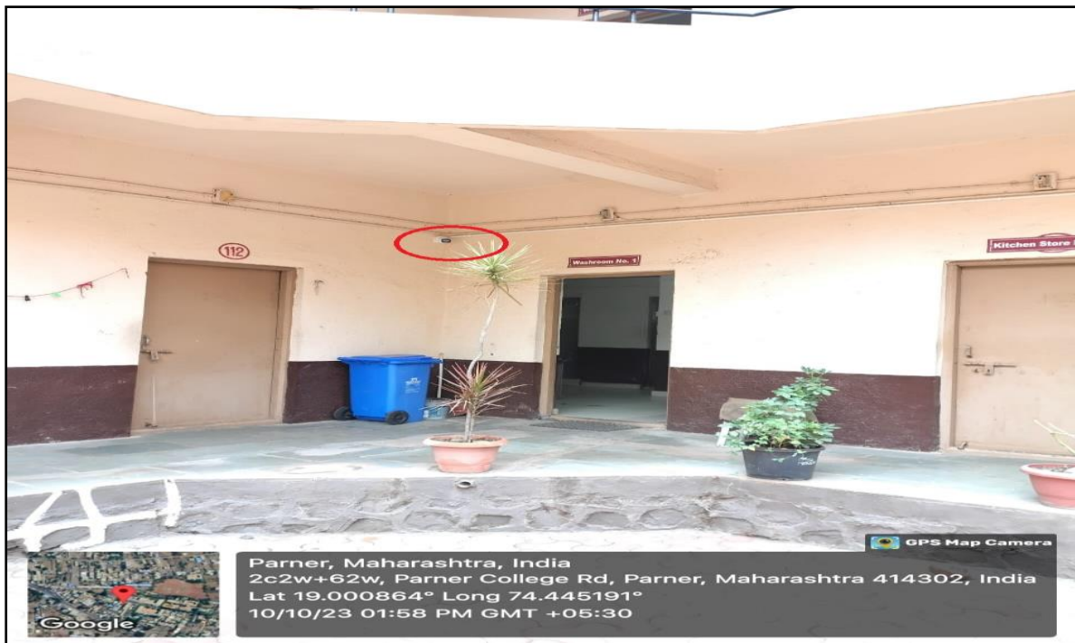
Picture 2: CCTV Surveillance System at Rajmata Jijau Girl's hostel
