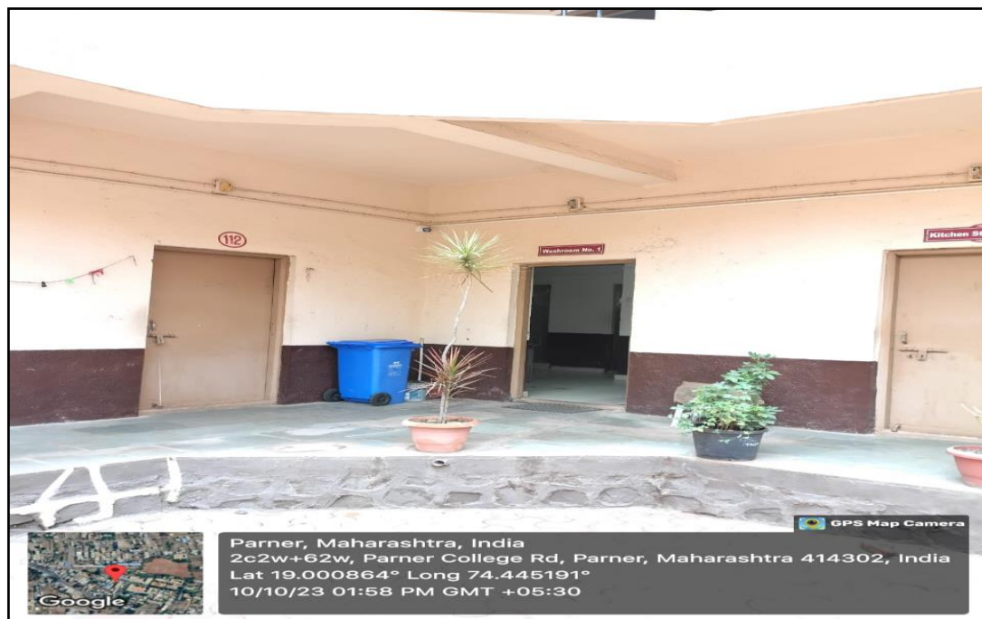
Picture 12: Washroom Facilities for Ladies at Rajmata Jijau Girl's hostel
