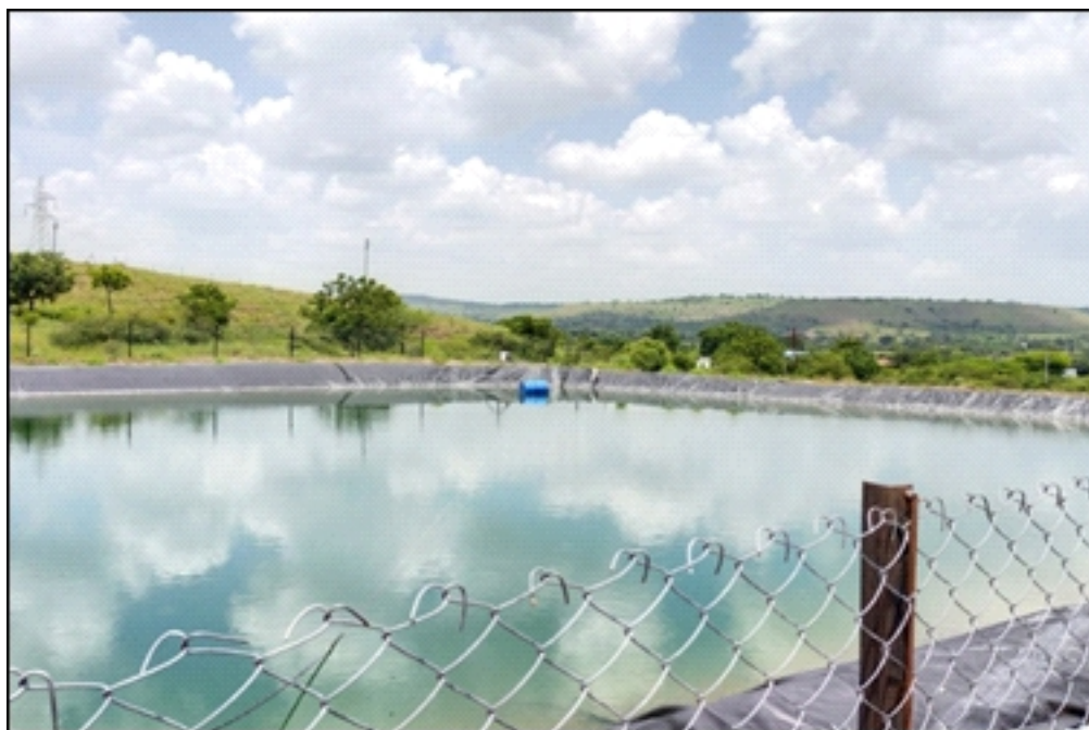
Figure No. 4: Farm pond with Poly-ethane (PE) lining and Galvanized Iron chain link fencing Conclusion:
