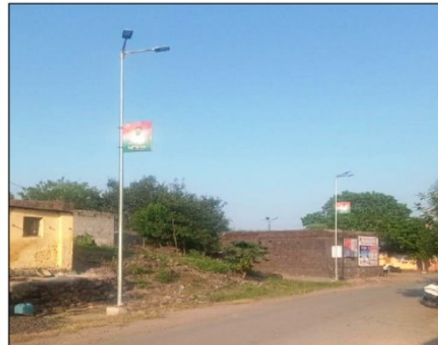
Picture 3: Pictures of Streetlight from karandi village
