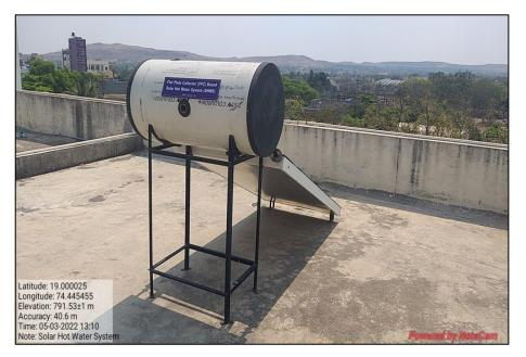
Picture 11: Solar water heater (FPC based) at Science Building
