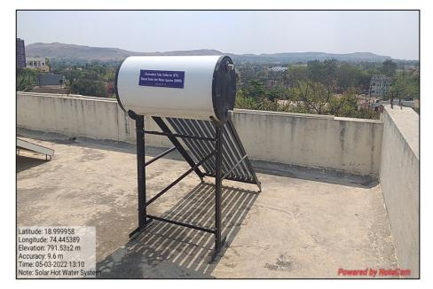
Picture 12: Solar water heater (ETC based) at Science Building
