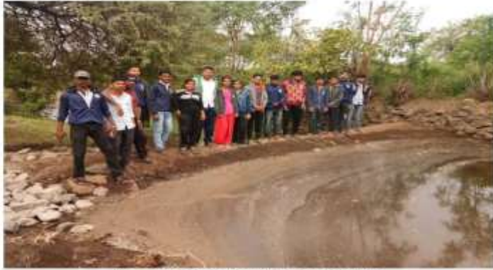
An earth dam built by volunteers.
