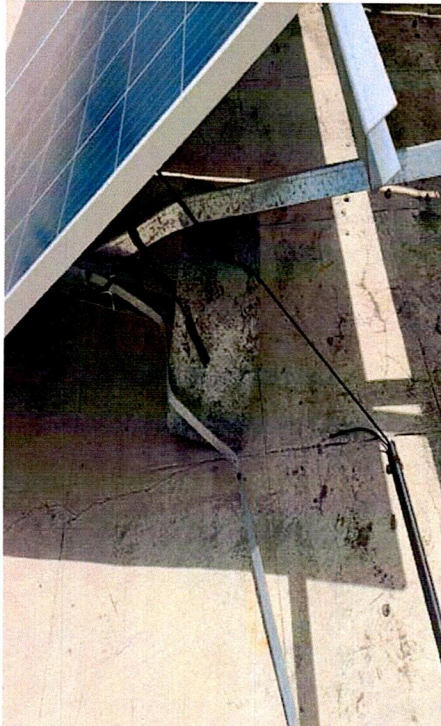
Open connections observed in wire.
