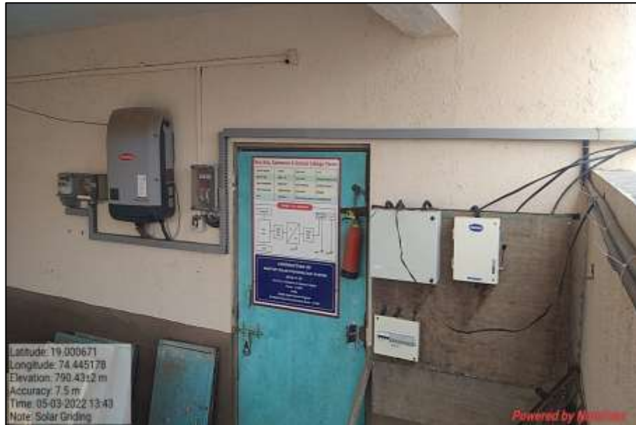
Picture 9: Solar Energy wheeled to grid panel at Arts and Commerce Building
