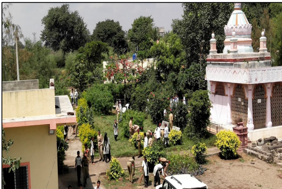
Picture 63: Mass Mobilization for construction of compost pits Date: 25/09/2018
