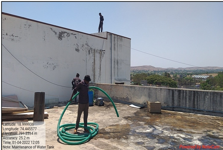
Picture 48: Cleaning and Maintenance of Water Tank
