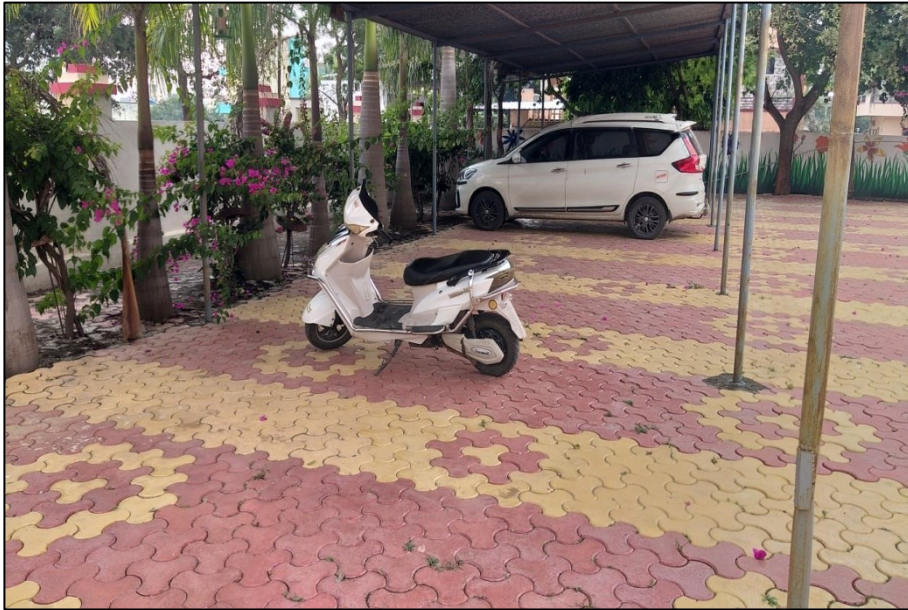
Picture 79: Parking reserved for Divyangjan
