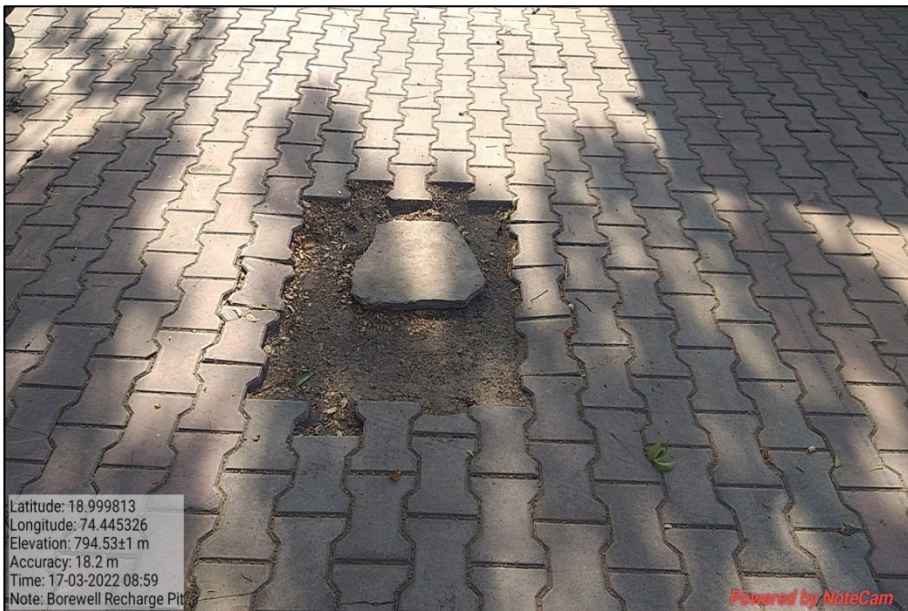
Picture 42: Bore well Recharge Pit
