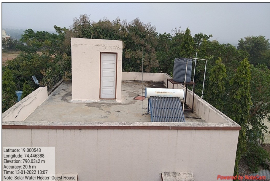
Picture 6: Solar water heater at Guest House
