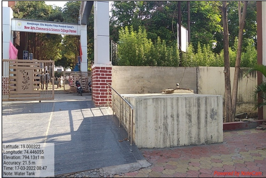
Picture 43: Water Tank
