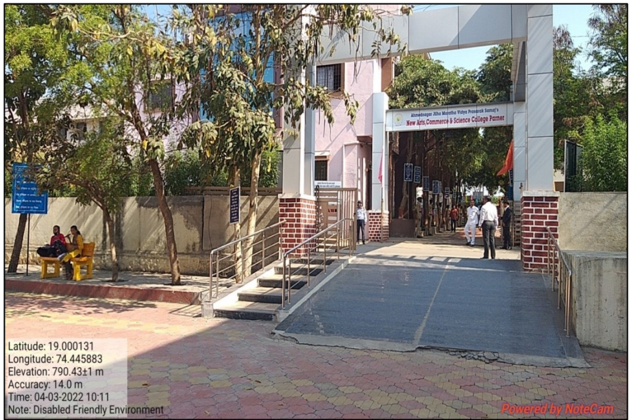
Picture 77: Ramp and Railings
