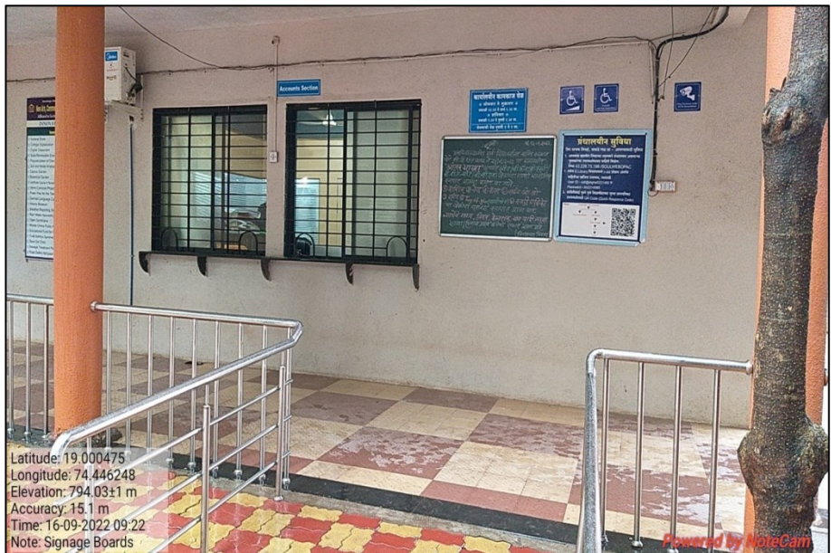
Picture 78: Ramp and Railings
