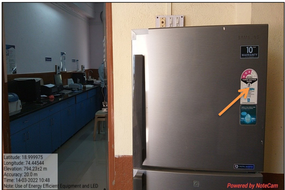
Picture 18: Use of Energy Efficient Equipments
