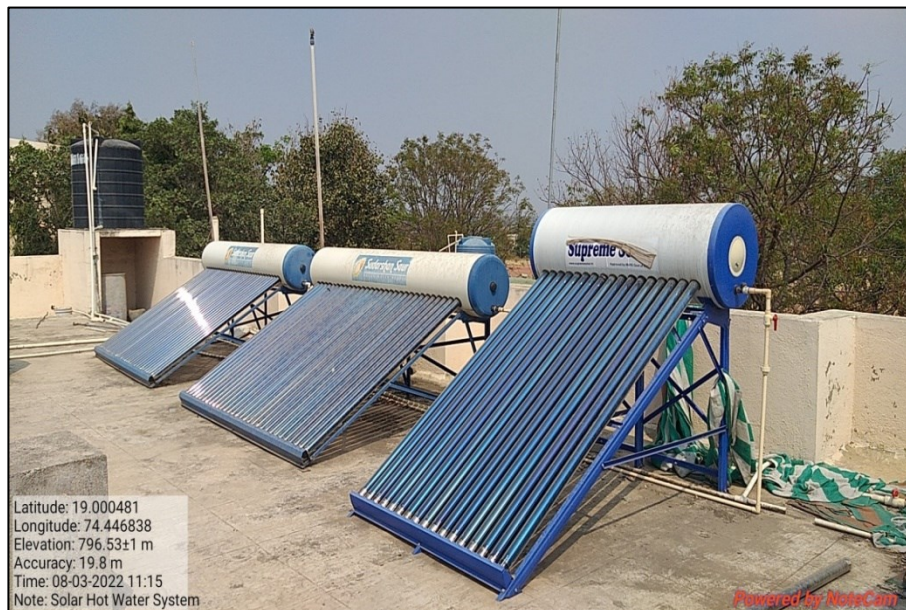
Picture 7: Solar water heater at Rajmata Jijau Girl’s hostel
