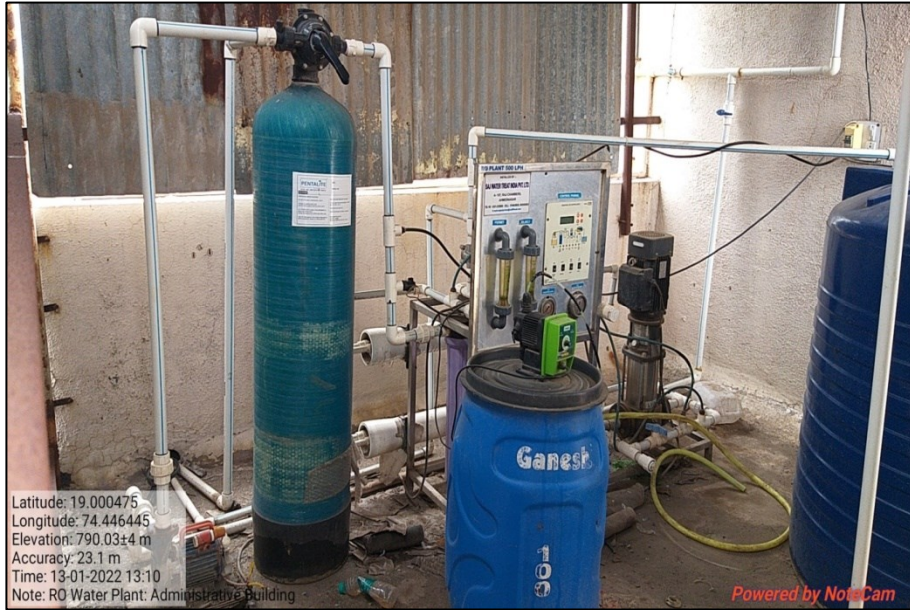
Picture 45: Water Purification Plant
