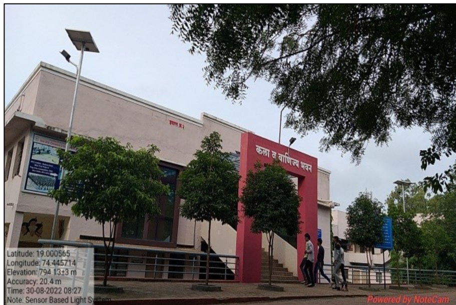
Picture 23: Sensor Based Energy Conservation through Street Lights
