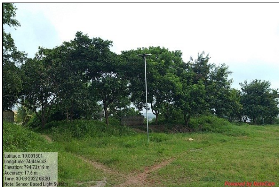
Picture 24: Sensor Based Energy Conservation through Street Lights
