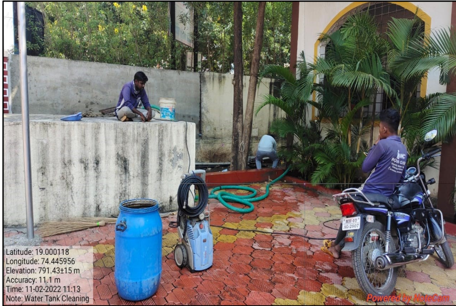
Picture 49: Cleaning and Maintenance of Water Tank
