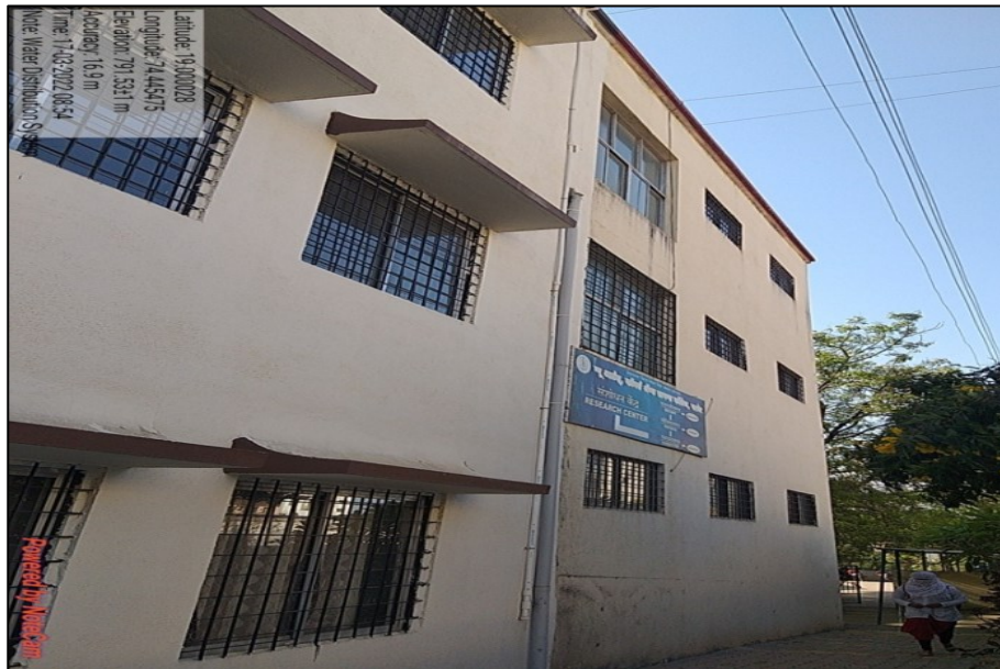
Picture 50: Water Distribution System
