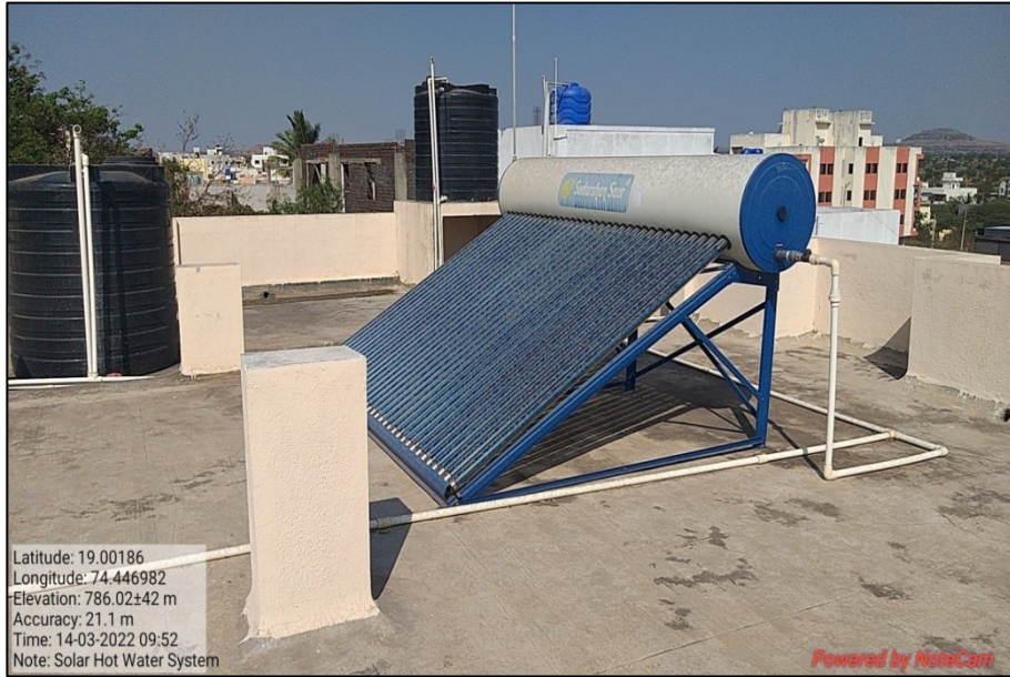
Picture 9: Solar water heater at boy's hostel
