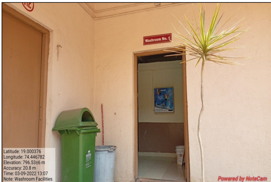
Picture 98: Washroom Facilities for Ladies at Rajmata Jijau Girl's hostel
