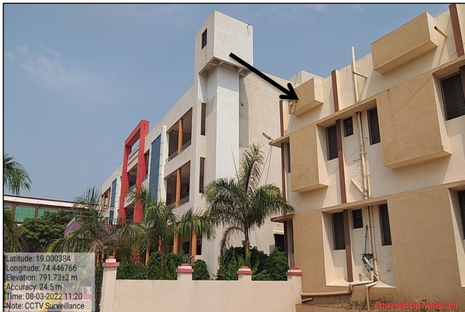
Picture 84: CCTV Surveillance System at Rajmata Jijau Girl’s hostel
