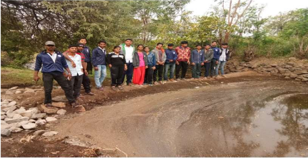
An earth dam built by volunteers.
