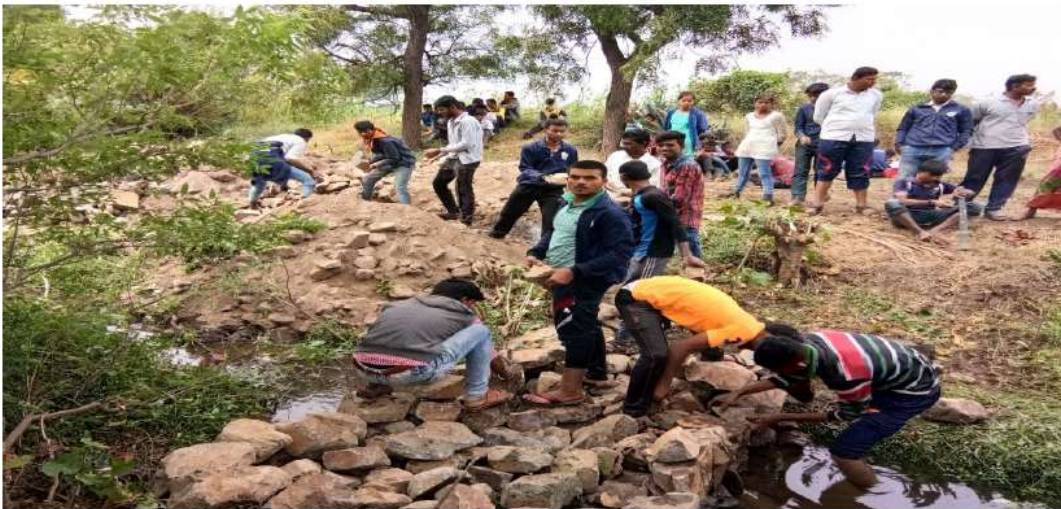
Volunteers building a stone and earth dam.
