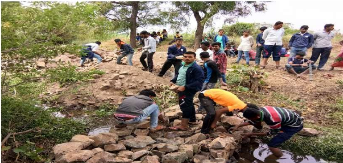
Volunteers building a stone and earth dam.
