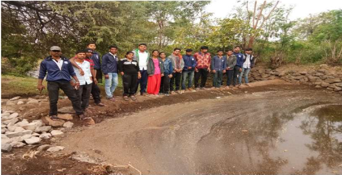
An earth dam built by volunteers.
