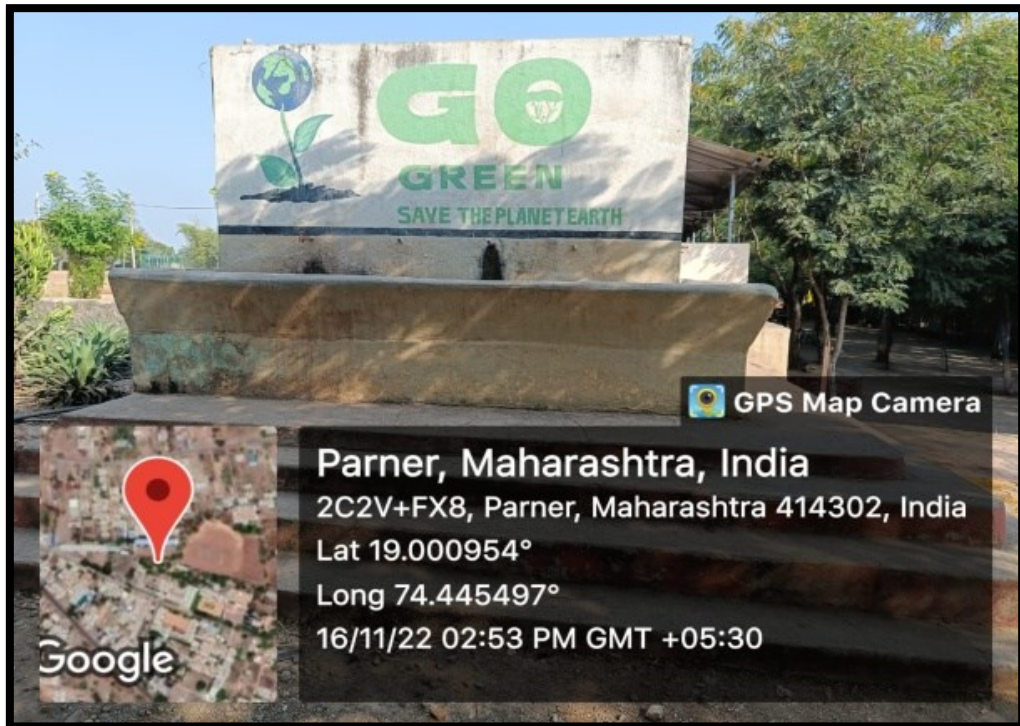
Water Tank in front of Arts & Commerce building
