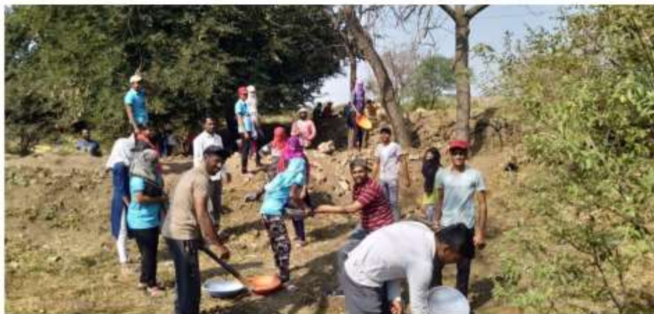
Volunteers building an earthen dam at a winter camp
