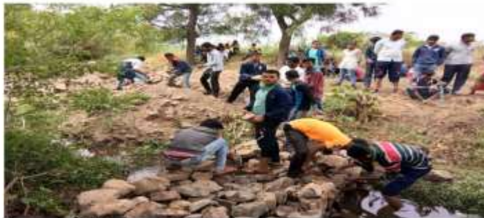
Volunteers building a stone and earth dam.
