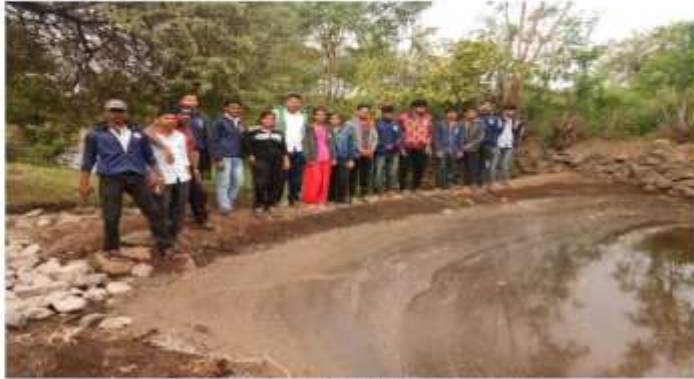
An earth dam built by volunteers.
