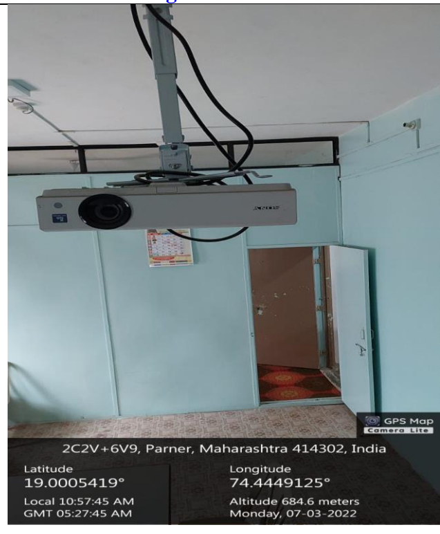
Arts & Com. Building Library
