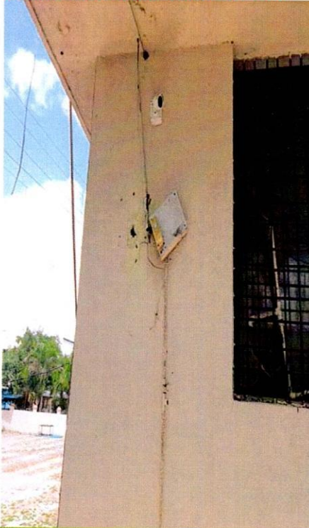
Open connections observed in wire.
