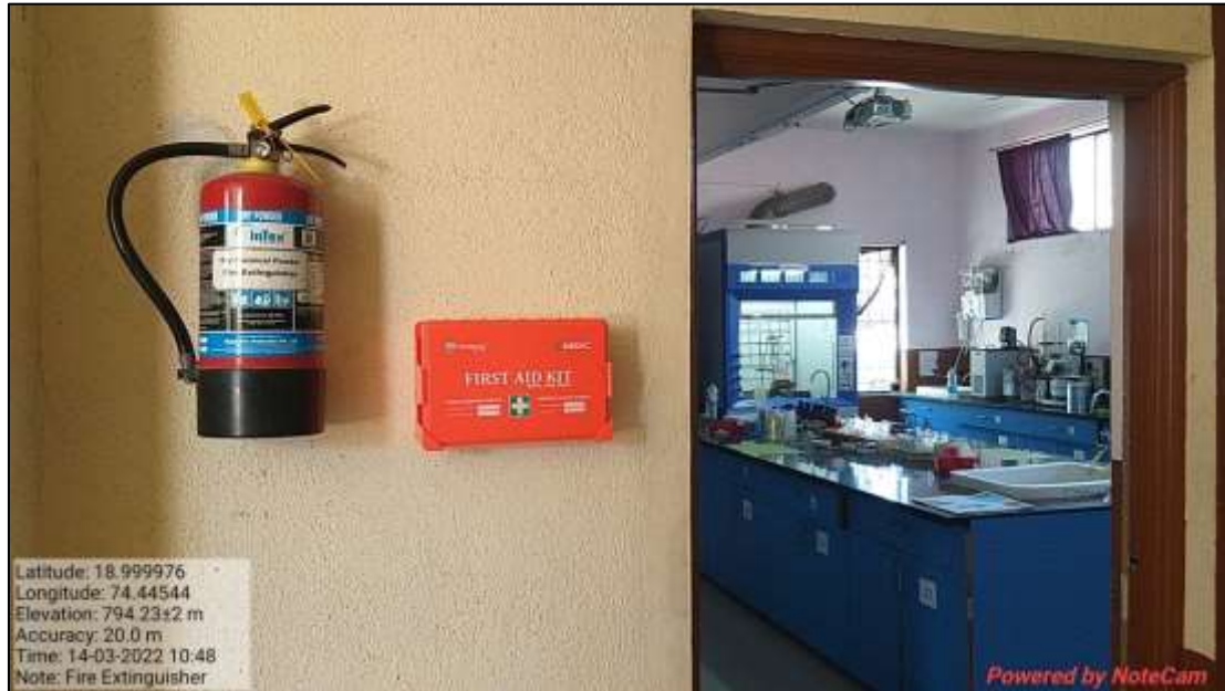
Figure 19 : Laboratory Safety (First Aid Box and Fire Extinguisher)
