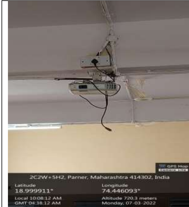
Science Building Classroom No. R-101
