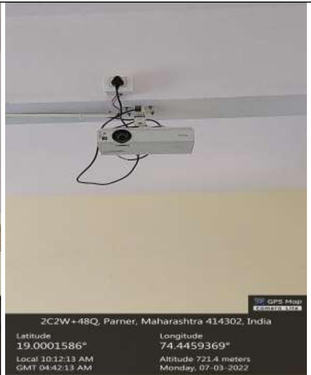
Science Building Classroom No. R-203
