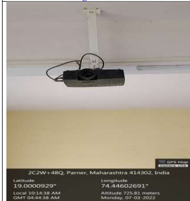
Science Building Classroom No. R-301
