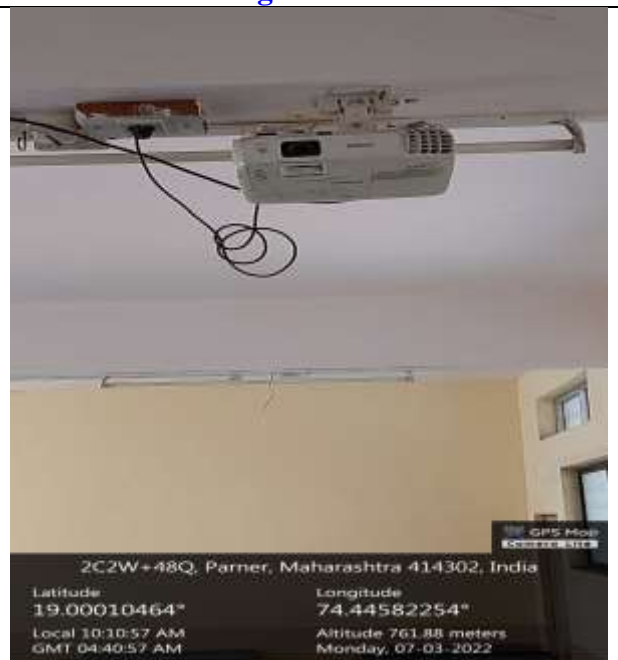
Science Building Classroom No. R-201
