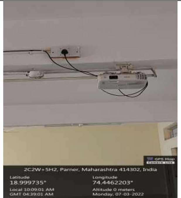
Science Building Classroom No. R-102
