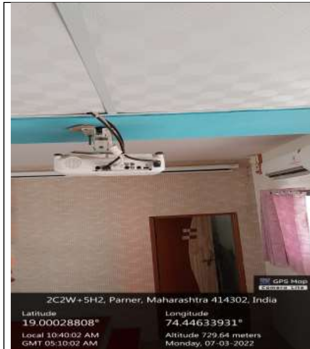
Administrative Building Conference Hall
