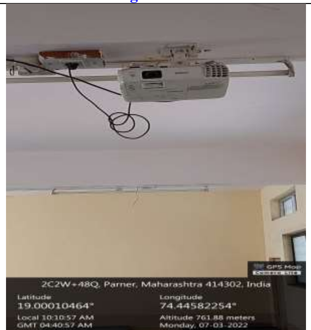
Science Building Classroom No. R-201
