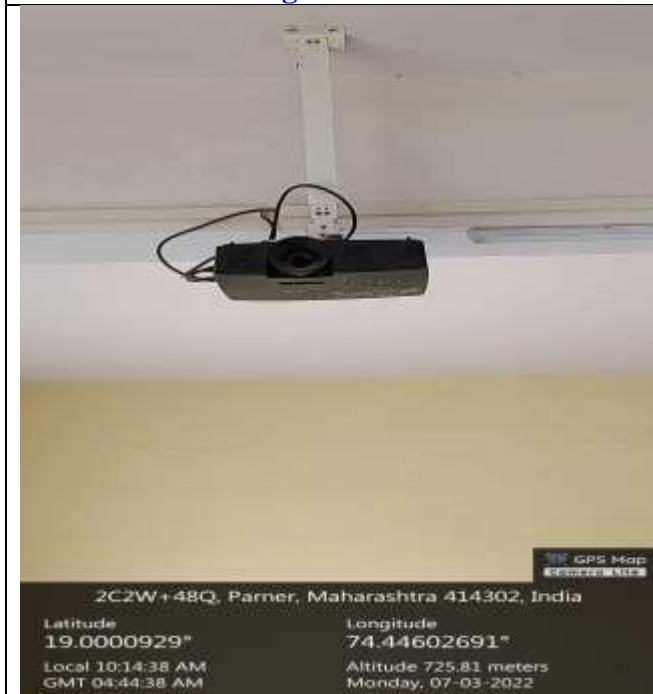
Science Building Classroom No. R-301
