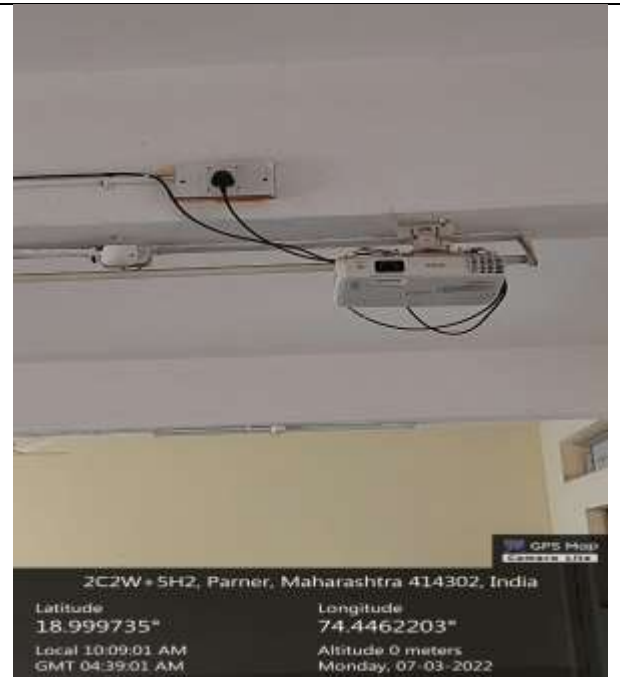
Science Building Classroom No. R-102
