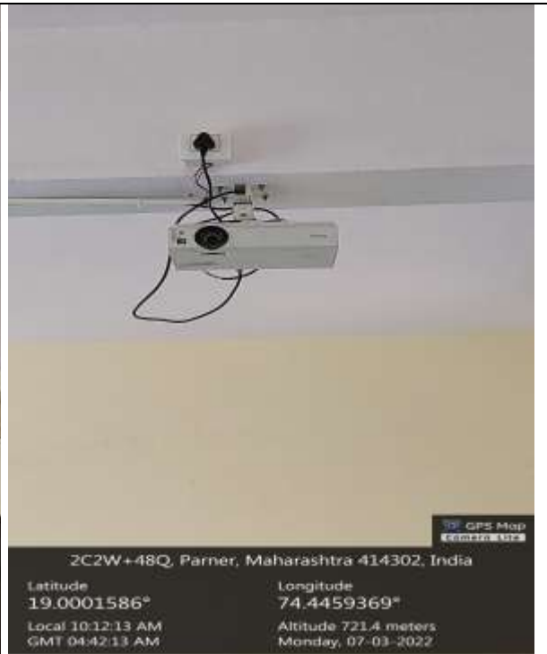
Science Building Classroom No. R-203
