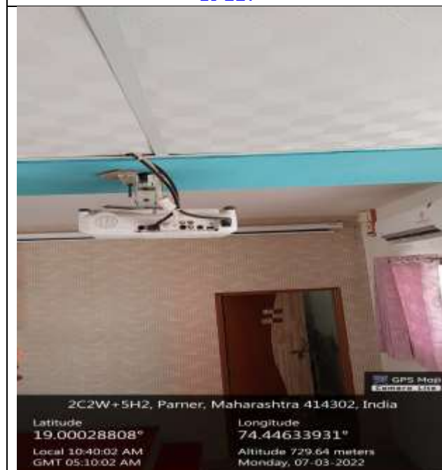
ADMIN Building Conference Hall
