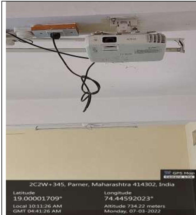
Science Building Classroom No. R-202
