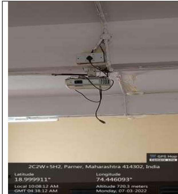
Science Building Classroom No. R-101
