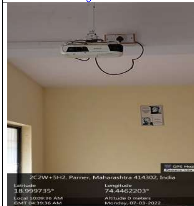
Science Building Classroom No. R-103
